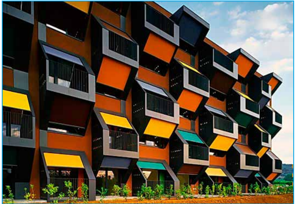
Housing Complex in Slovenia is a Series of Honeycomb Modular Apartments by Inhabitat.com that uses solar shading and natural ventilation to regulate its interiors all year-round.
