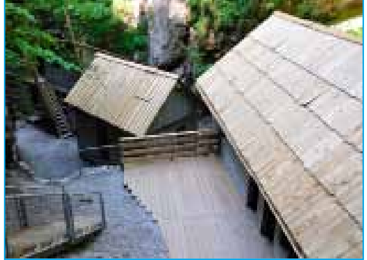
Washrooms and care facility.
