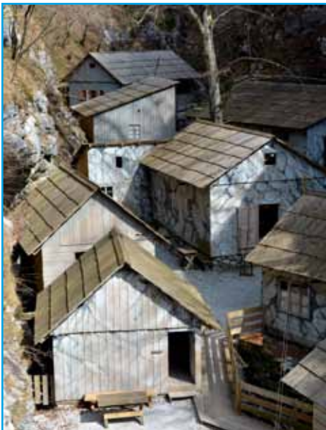
Franja Partisan Hospital in the Pasice gorge.
