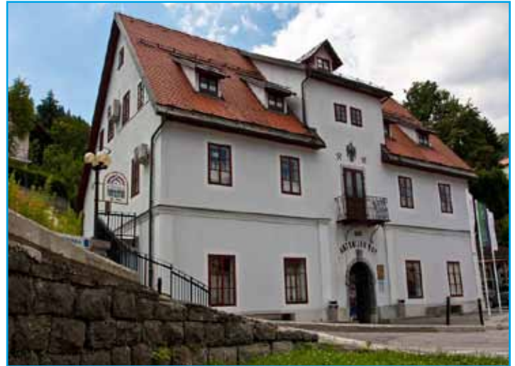
Entrance to Anthony's shaft.
