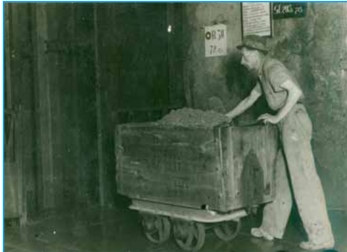
Transport of ore to level XI of the mine.
